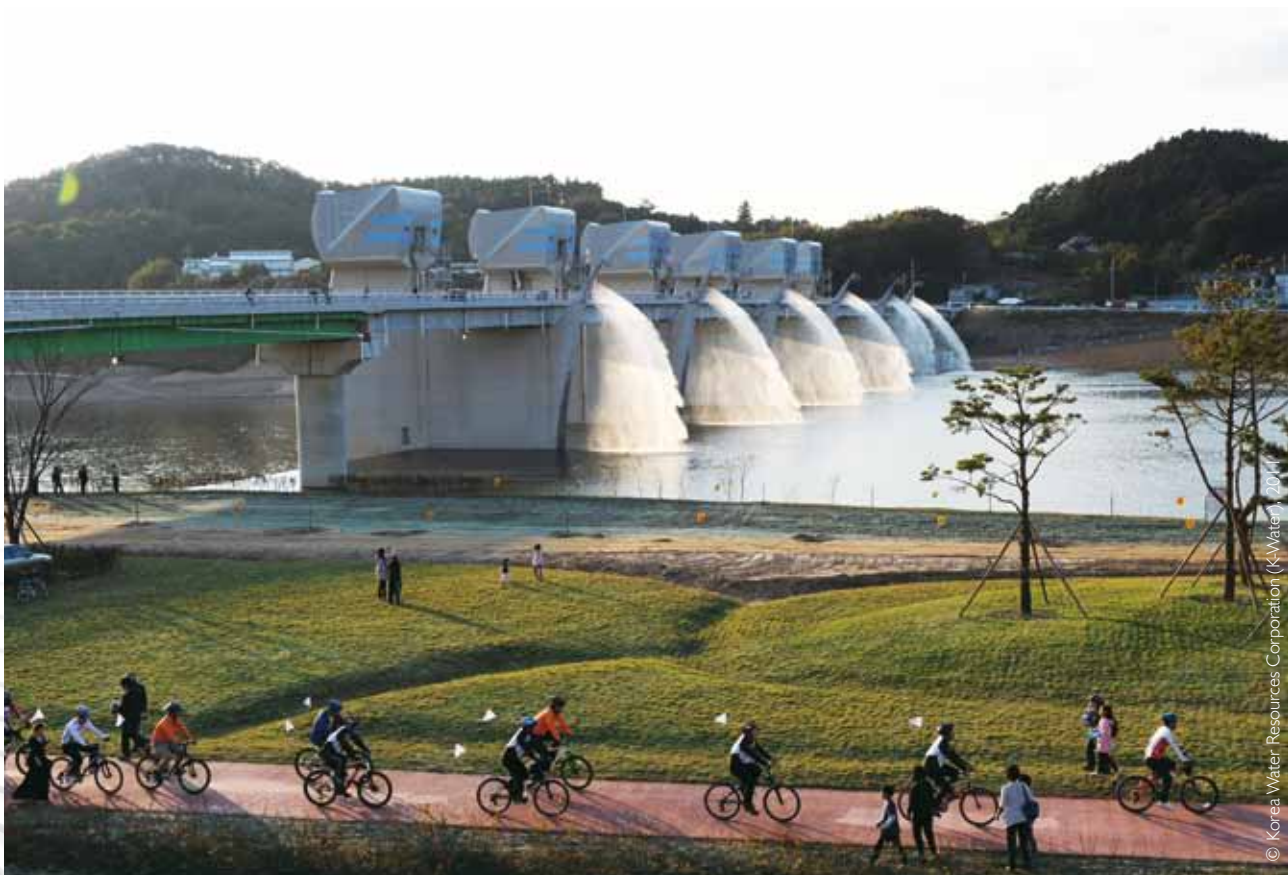
Four Major Rivers Restoration Project.
