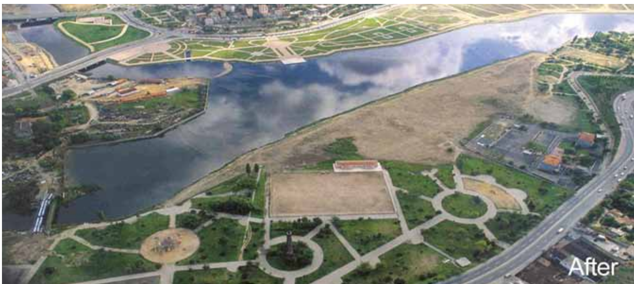
Cleaning up a polluted urban waterway became the catalyst for multi-dimensional economic & social development in Istanbul
